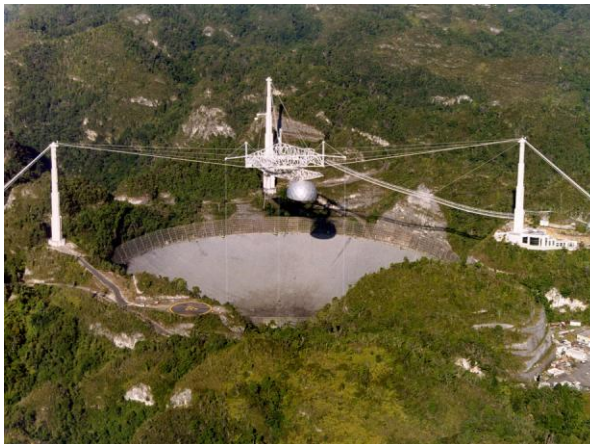
An image of the Arecibo Radio Telescope in Puerto Rico. The Gregorian dome, which houses the main suite of research instruments, and its suspension structure are visible over the main reflector below. Credit: Arecibo Observatory/NSF.
