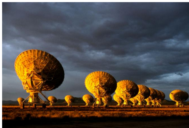
The Very Large Array (VLA) telescope, located about 80 km west of Socorro, NM, is composed of 27 individual antennas arranged in a "Y" pattern. In their closest configuration (about 1 km wide), the VLA is able to image large portions of the sky. In its largest configuration (about 36 km wide) the VLA is able to home in on the fine details of astronomical objects. Credit: Andrew Clegg, National Science Foundation.
