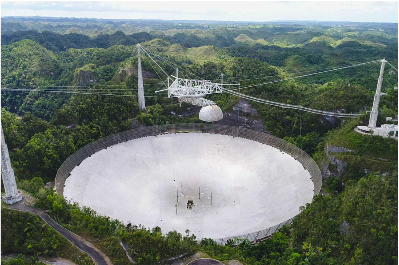
Figure 8: A bird's-eye view of the massive, 1000-foot diameter radio dish.
