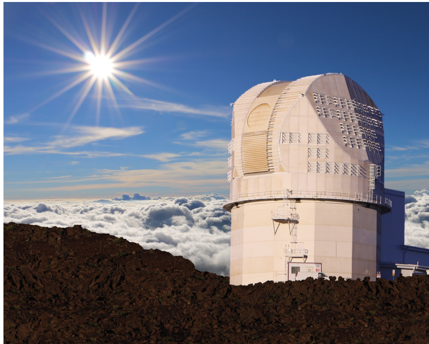
Figure 9: Nearly completed DKIST facility on the summit of Haleakala, Maui.
