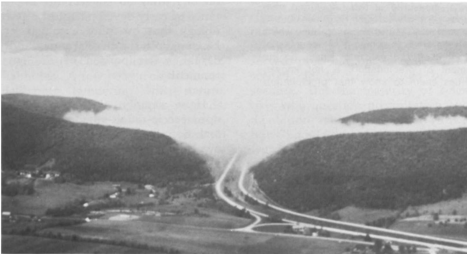
Figure VI-8 — A DRIVING HAZARD
